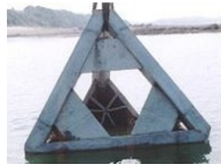
Regular trigonal pyramid type reef (3.1x3.1x2.9m)
